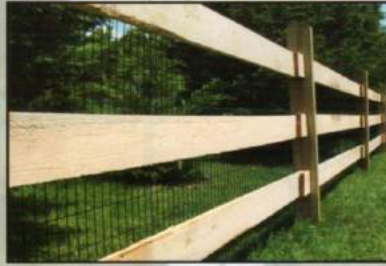
3 Rail Slip Board, 3" x 6" Treated Posts, 1" x 6" x 12' Hemlock Boards
